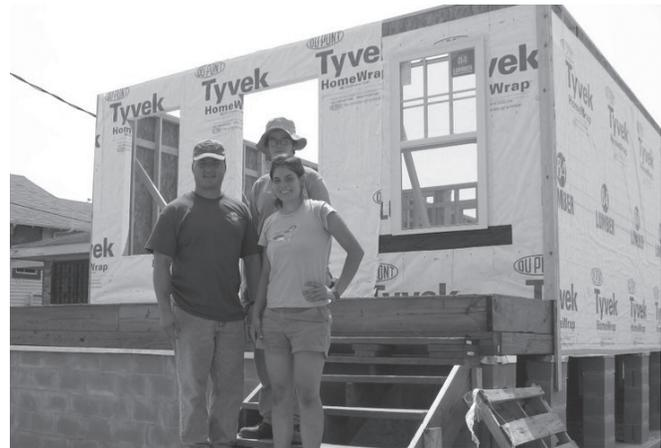
**BEFORE AND AFTER**--This is the house we worked on most of the day. The Tyvek was completed and chalk lines placed for the siding; Staples were hammered down; closets framed; flooring was leveled; and the yard was graded. On the right are our supervisors Emily and John.
