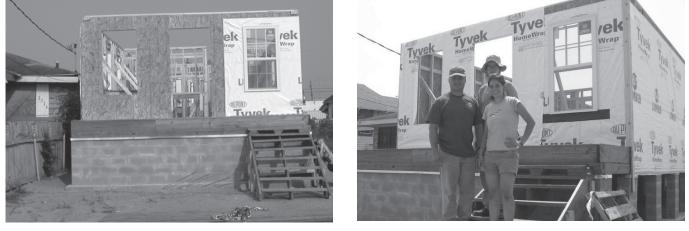
**BEFORE AND AFTER--**This is the house we worked on most of the day. The Tyvek was completed and chalk lines placed for the siding; Staples were hammered down; closets framed; flooring was leveled; and the yard was graded. On the right are our supervisors Emily and John.
